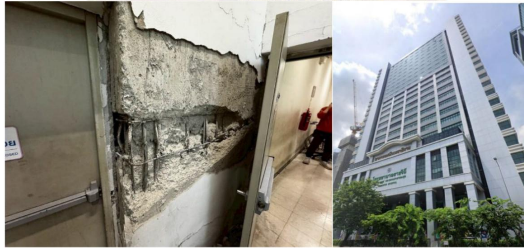
Fig. 15 Severe damage observed at shear wall including vertical bar buckling and concrete spalling in the lower stories of a 25-story building due to lack of seismic detailing with horizontal reinforcing bars of about 300 mm spacing
