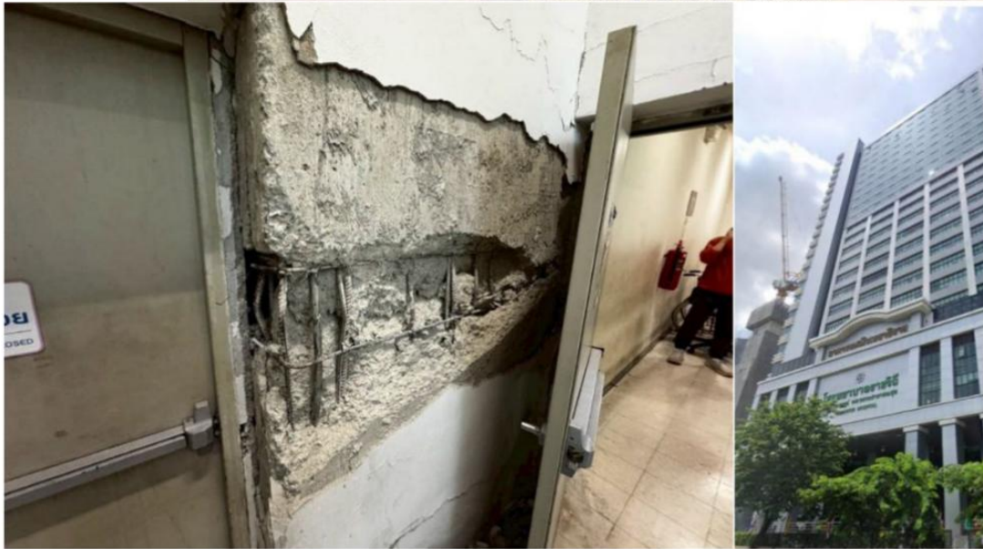
Fig. 15 Severe damage observed at shear wall including vertical bar buckling and concrete spalling in the lower stories of a 25-story building due to lack of seismic detailing with horizontal reinforcement of about 300 mm spacing
