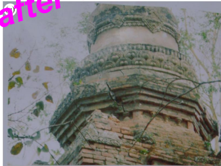
Figure 5. (a) Chedi Pasak before 2011 earthquake. (b) The schematic plot of Chedi Pasak in different layers. (c) Observed wide cracks at the lower top part. (d) Tilt could be clearly seen at the top spire following the 2011 earthquake in Myanmar located at 50 km to Chiang Saen. (Online version in colour.)
