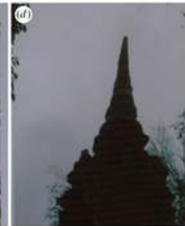
Figure 5. (a) Chedi Pasak before 2011 earthquake. (b) The schematic plot of Chedi Pasak in different layers. (c) Observed wide cracks at the lower top part. (d) Tilt could be clearly seen at the top spire following the 2011 earthquake in Myanmar located at 50 km to Chiang Saen. (Online version in colour.)
